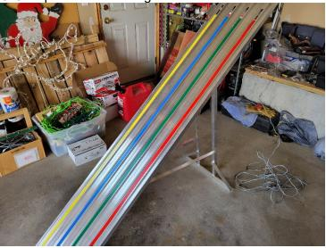
12. The last piece of the track (A-6) is the piece that stops the cars at the end of the race. This piece lines up differently and has no pins. Attach A-6 to the end of A-5 with C-Clamps by adjusting the clamp first, and setting it in place.
